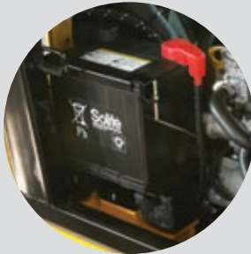
Rotational Battery Installation
